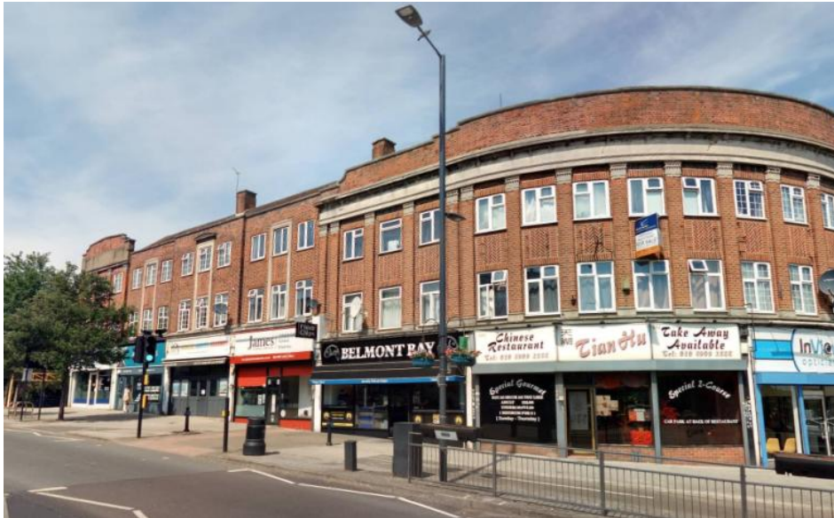
Views along Kenton Lane (West) from Belmont Circle
