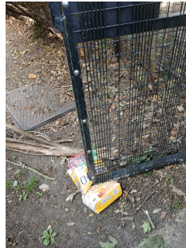
Gate propped open at rear of blk 14-25 Kipling
