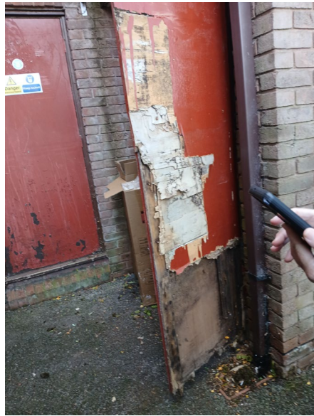
Damaged bin store door at rear of 1-9 fern house
