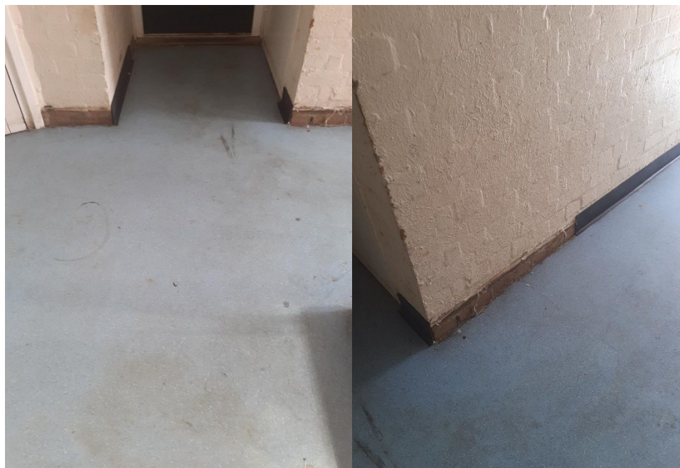
Lower Rd – Skirtings board missing in areas
