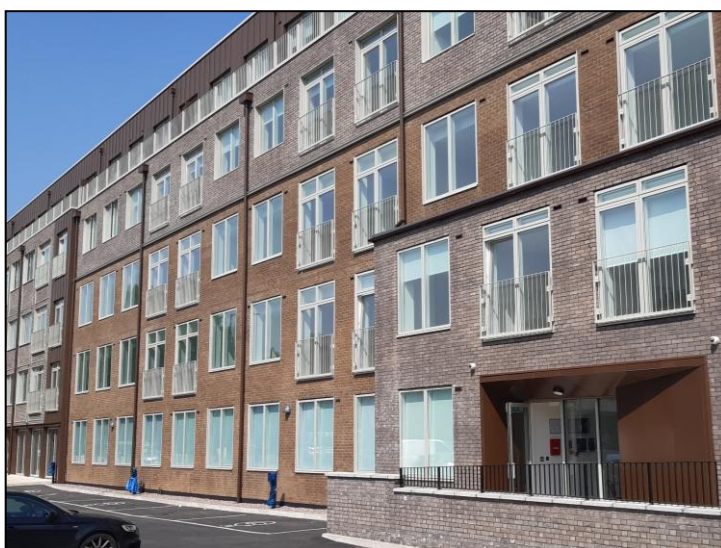
Stewart House, 414-436 Kenton Road, Harrow
