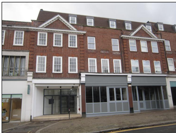
29A Bridge Street, Pinner
