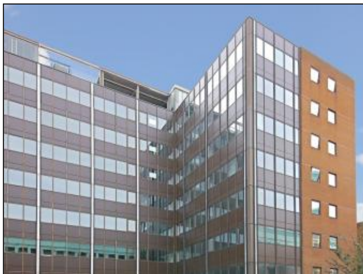
Queens House, Kymberley Road, Harrow
