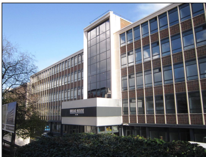
Broad House, 175-205 Imperial Drive, Rayners Lane
