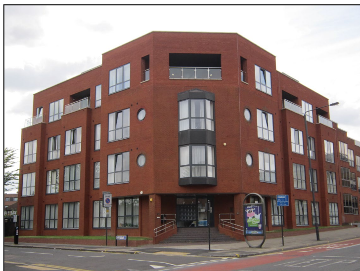
Kirkfield House, 118 Station Road, Harrow
