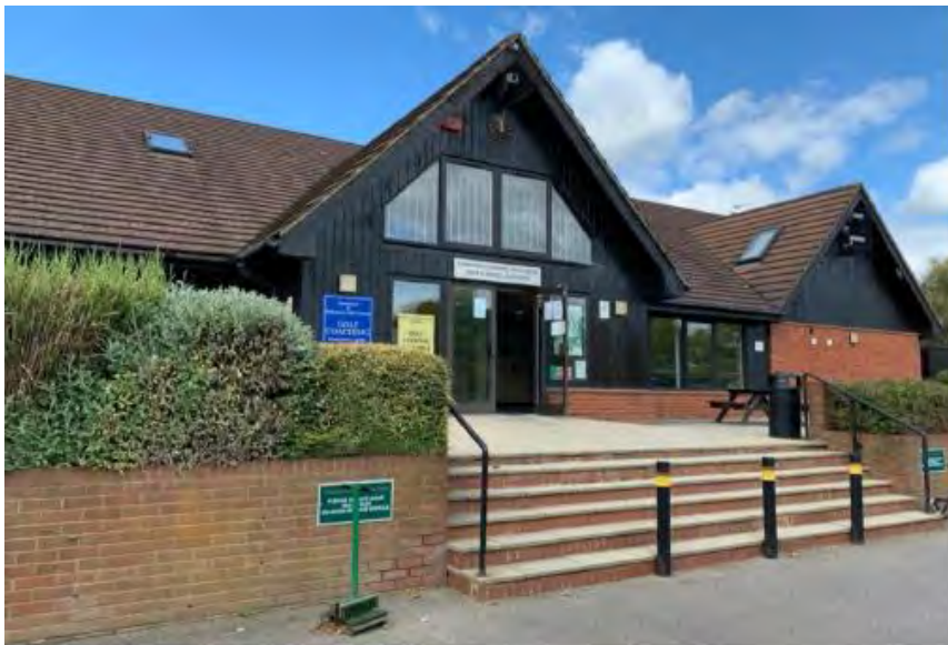
Above & Below: Photograph showing former clubhouse building
