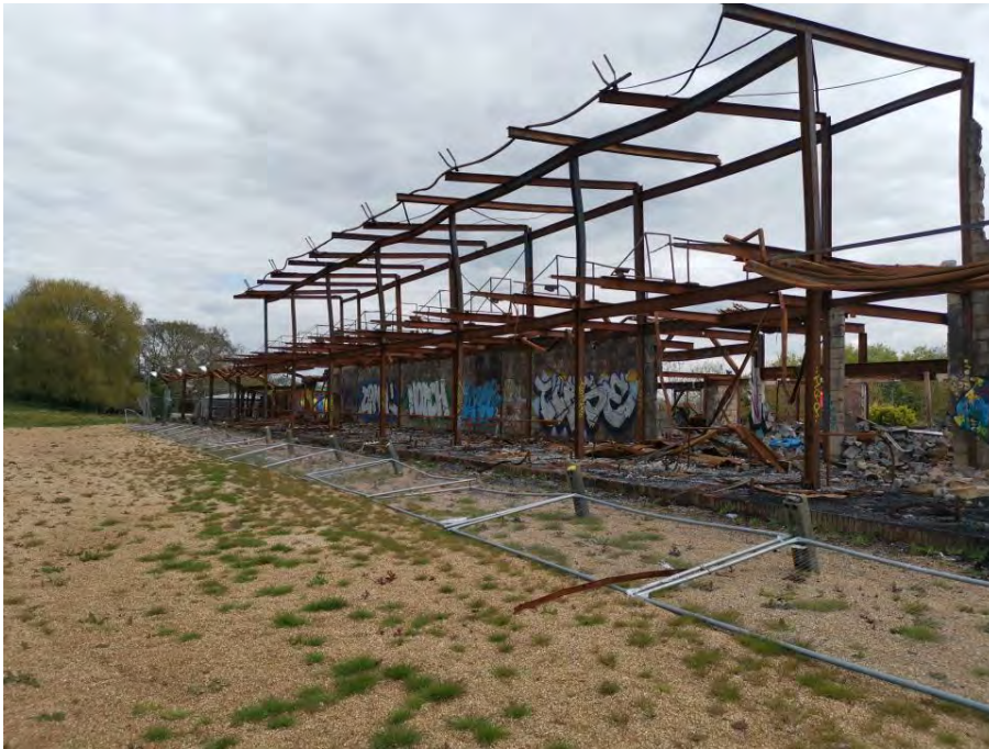
Above: Existing remaining structure
