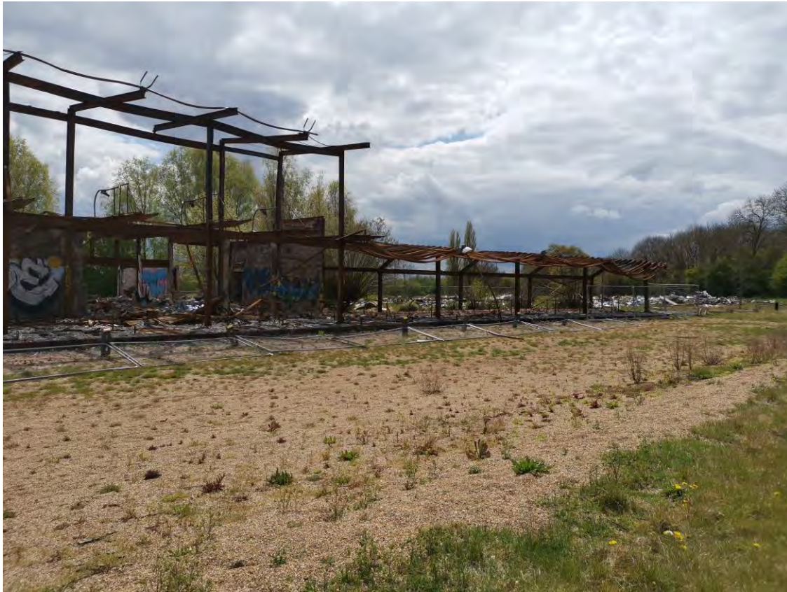
Above/Below: Former front elevation of the remaining structure from the northern side of the site
