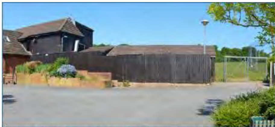
Image 3: Brick walls and timber fencing associated with the building
