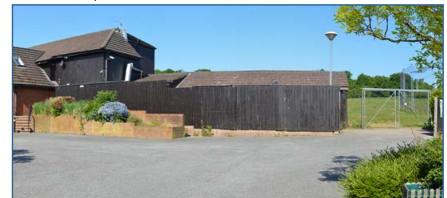
Image 3: Brick walls and timber fencing associated with the building
