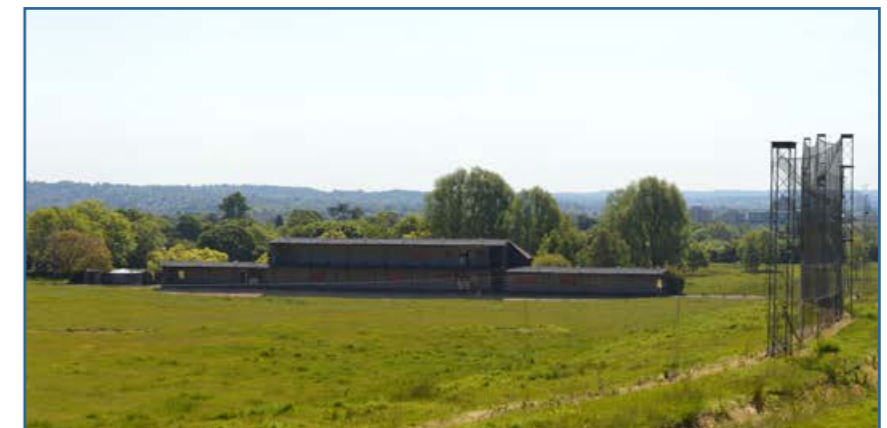
Image 2: Existing building as viewed from the upper slopes of the site
