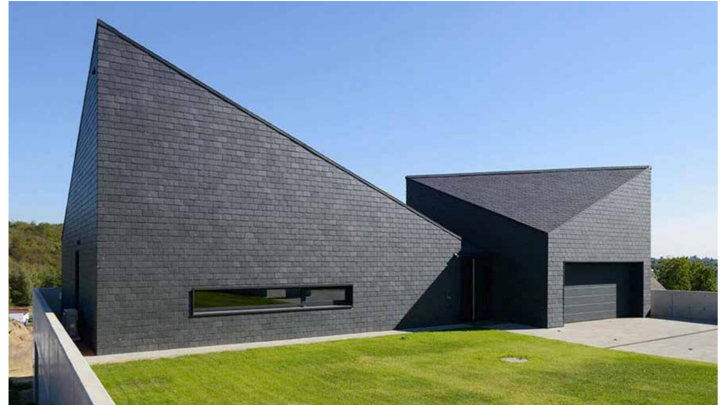
2 - Modern slate cladding with crisp edge detailing and matching coping details - Credit: RS+ Architects
