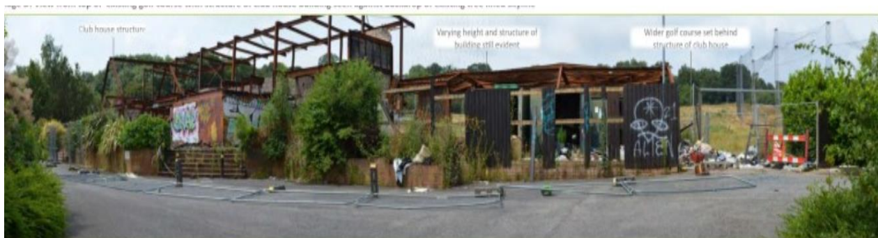
Image F: Damaged clubhouse building
