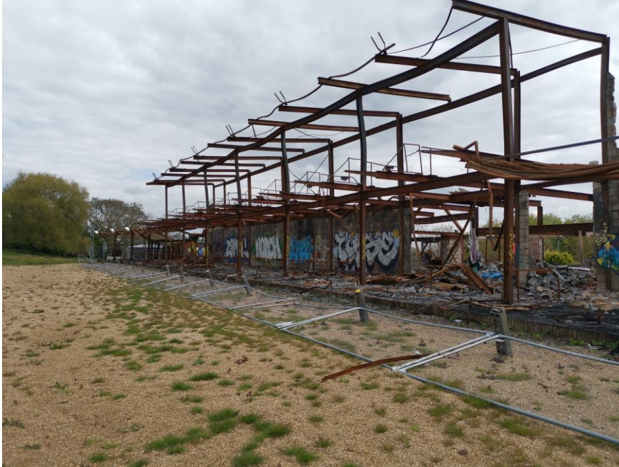
Above: Existing remaining structure
