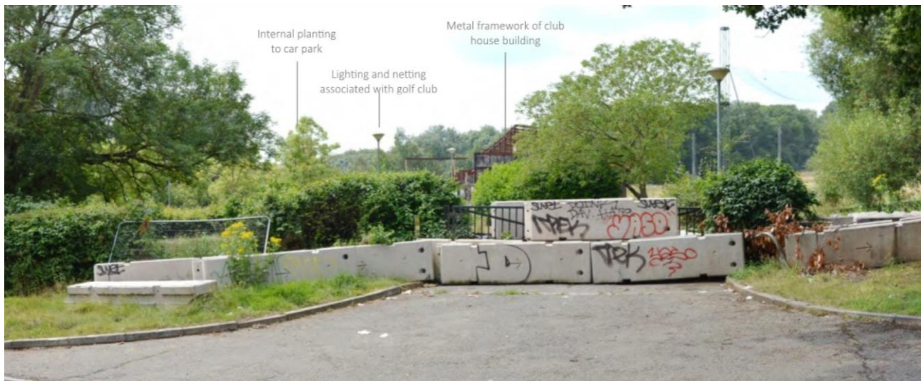
Existing View of Site from eastern entrance along Brockley Hill with security gate.
