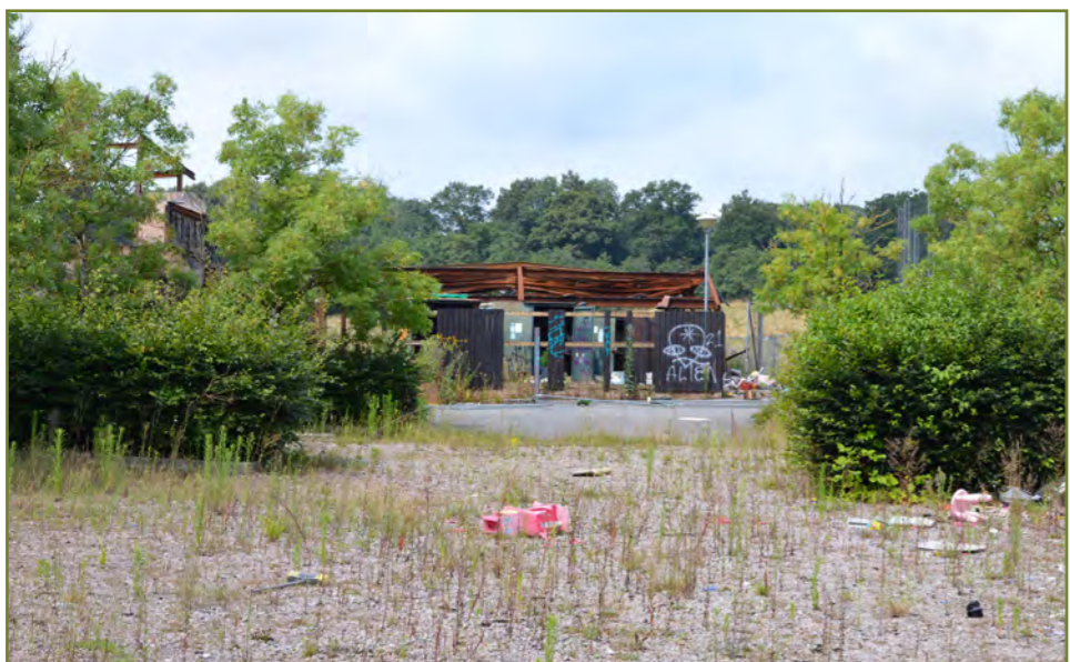
Image J: Areas of hardstanding in car parking
