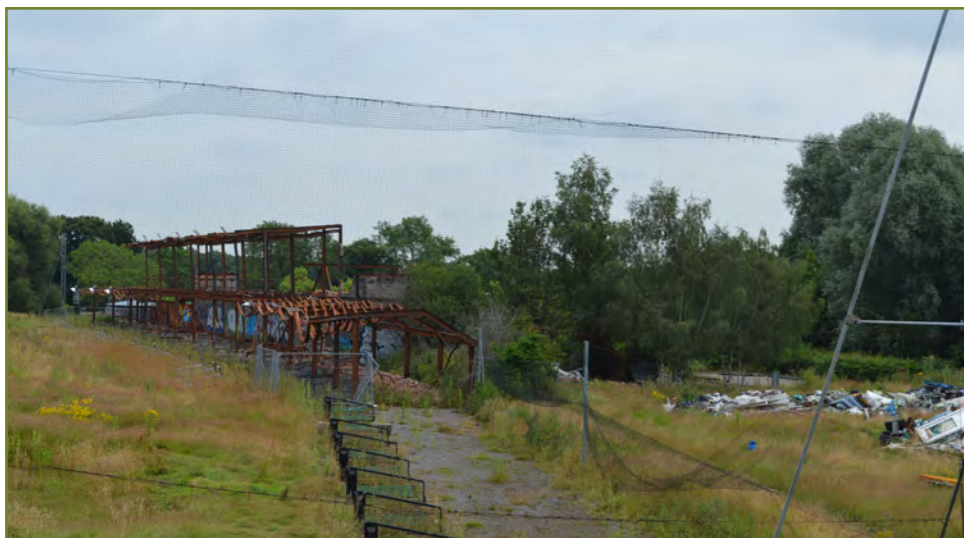
Image I: Areas of hardstanding adjacent to wings of club house
