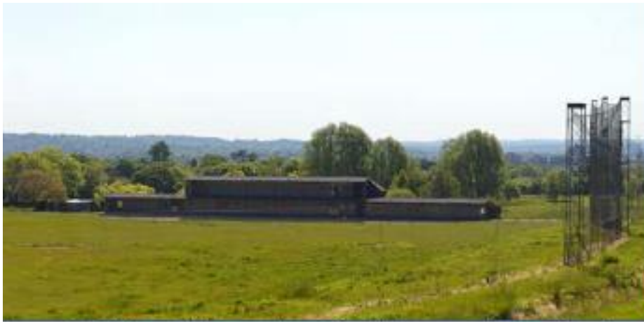
Image 2: Existing building as viewed from the upper slopes of the site Above: Former Club House building in views from the north
