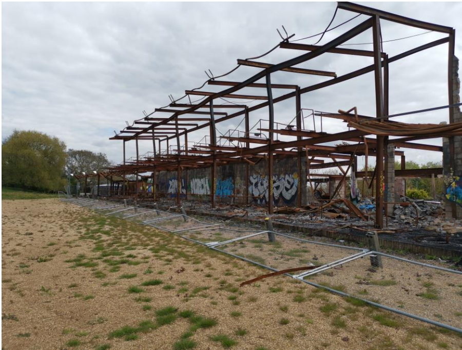
Above: Existing remaining structure
