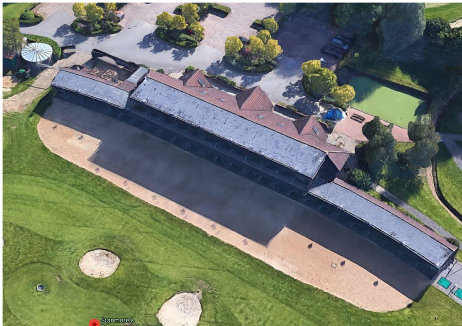
Above: Aerial view of building and developed curtilage pre fire
