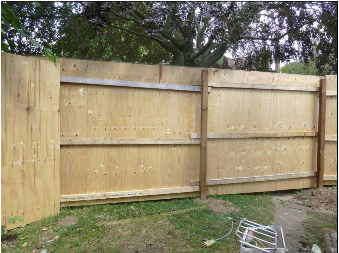
Photograph F – Example of Timber Hoarding Tree Protective Fencing.
