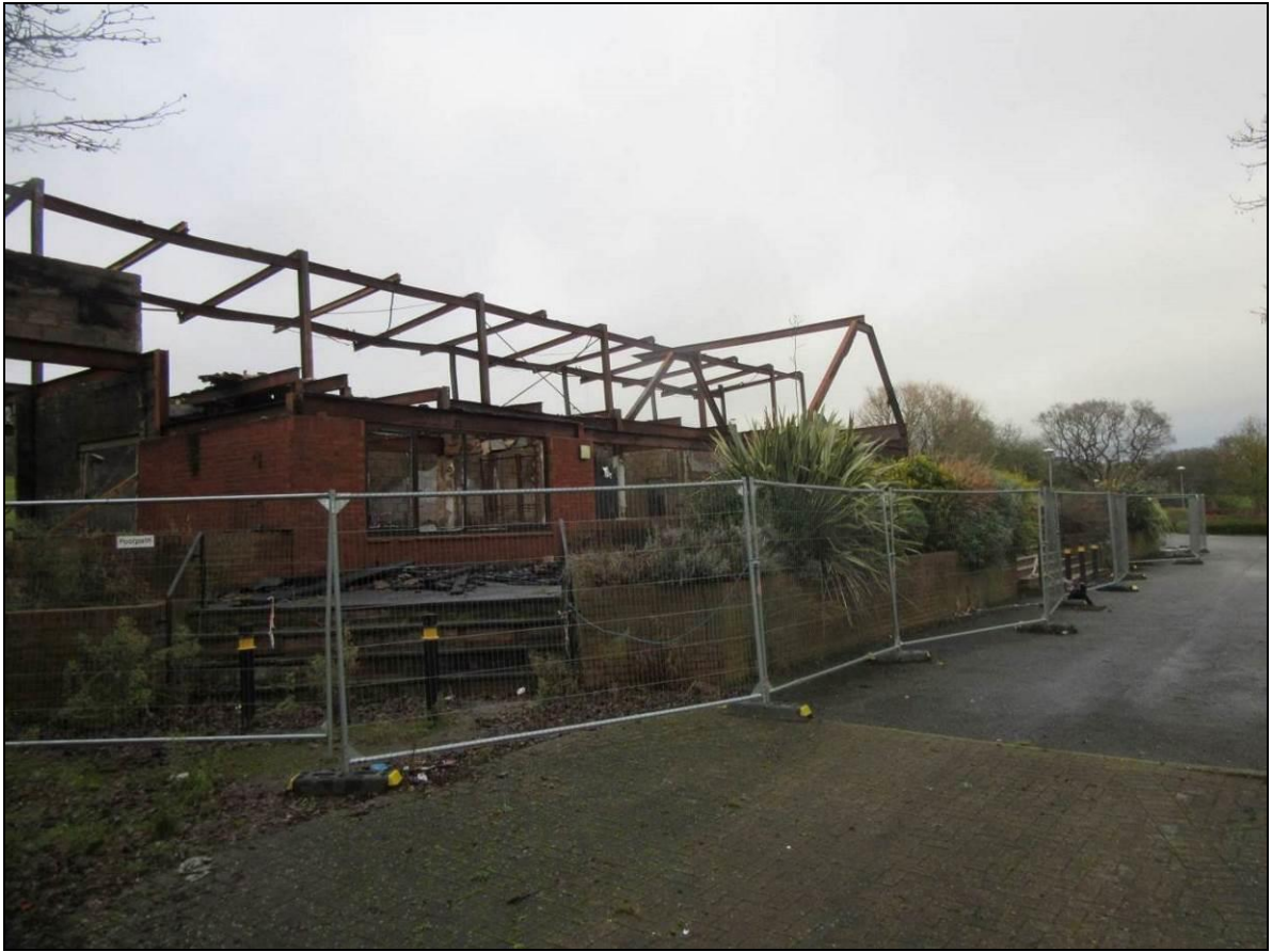
Photograph A – Showing the remnants of the existing building.
