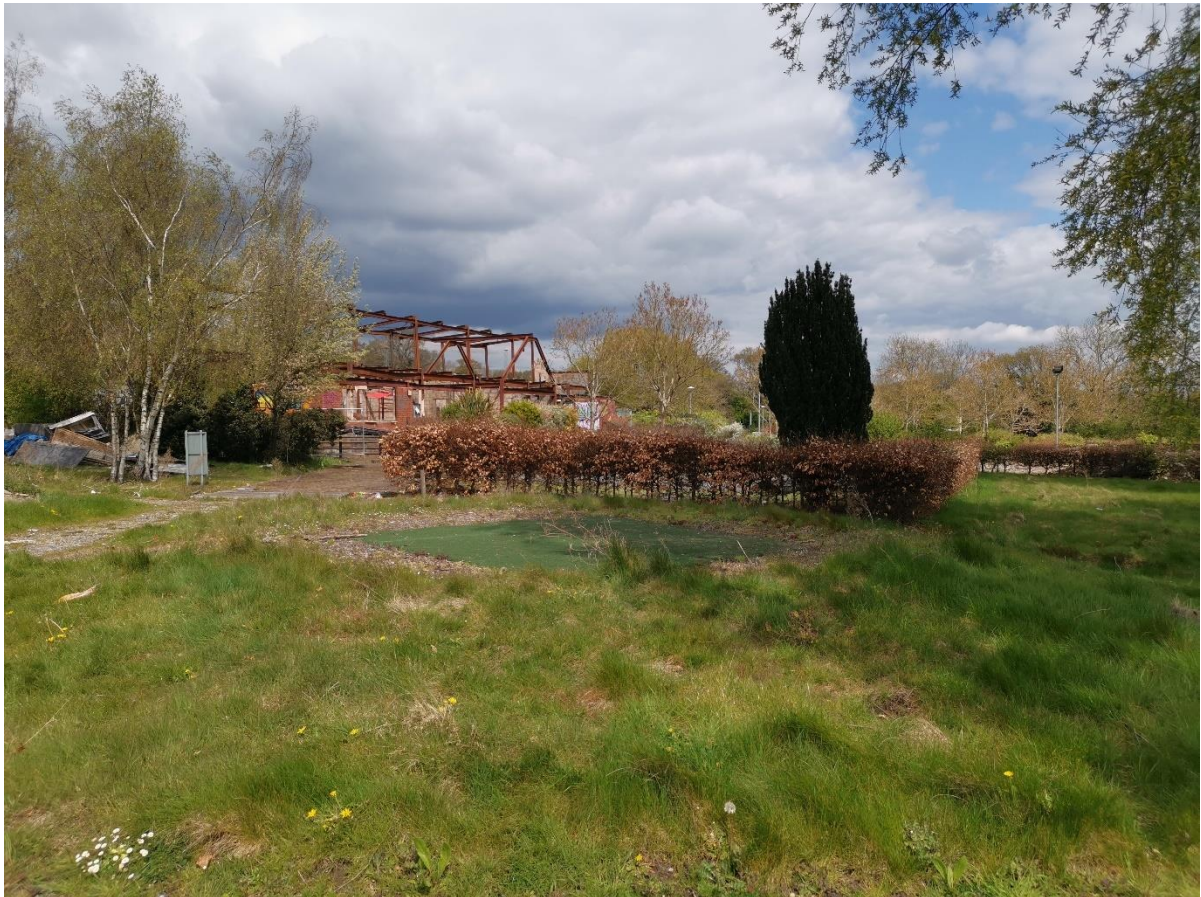
Figure 17: View from southern side of the site
