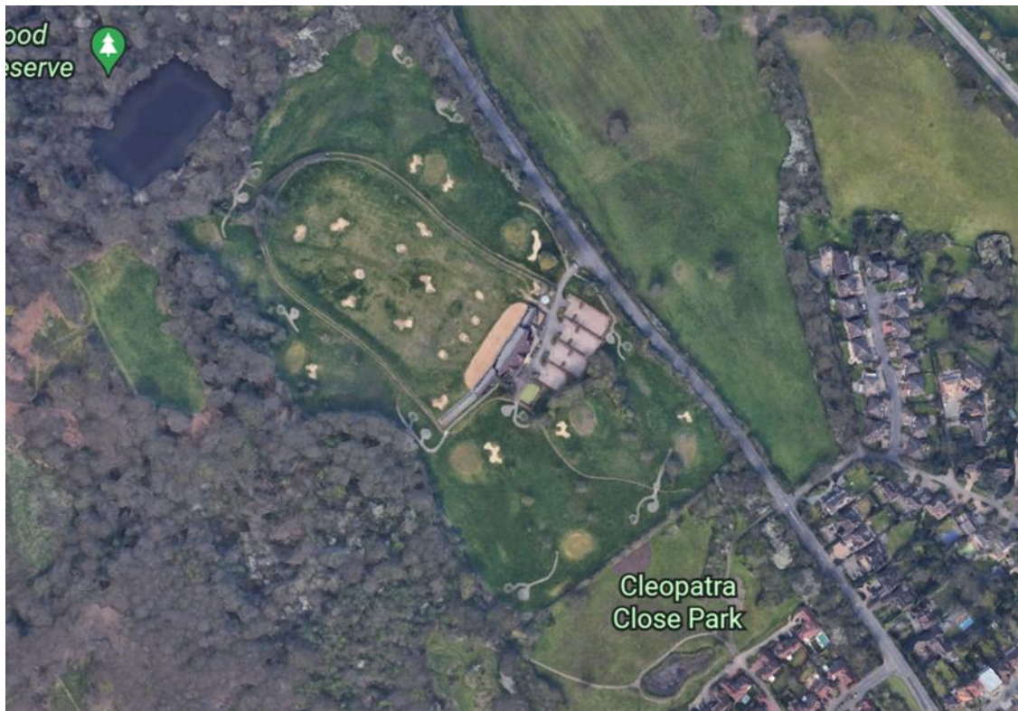
Figure 11: Aerial photograph of site and its context from Google Earth (Please note this image is prior to fire)
