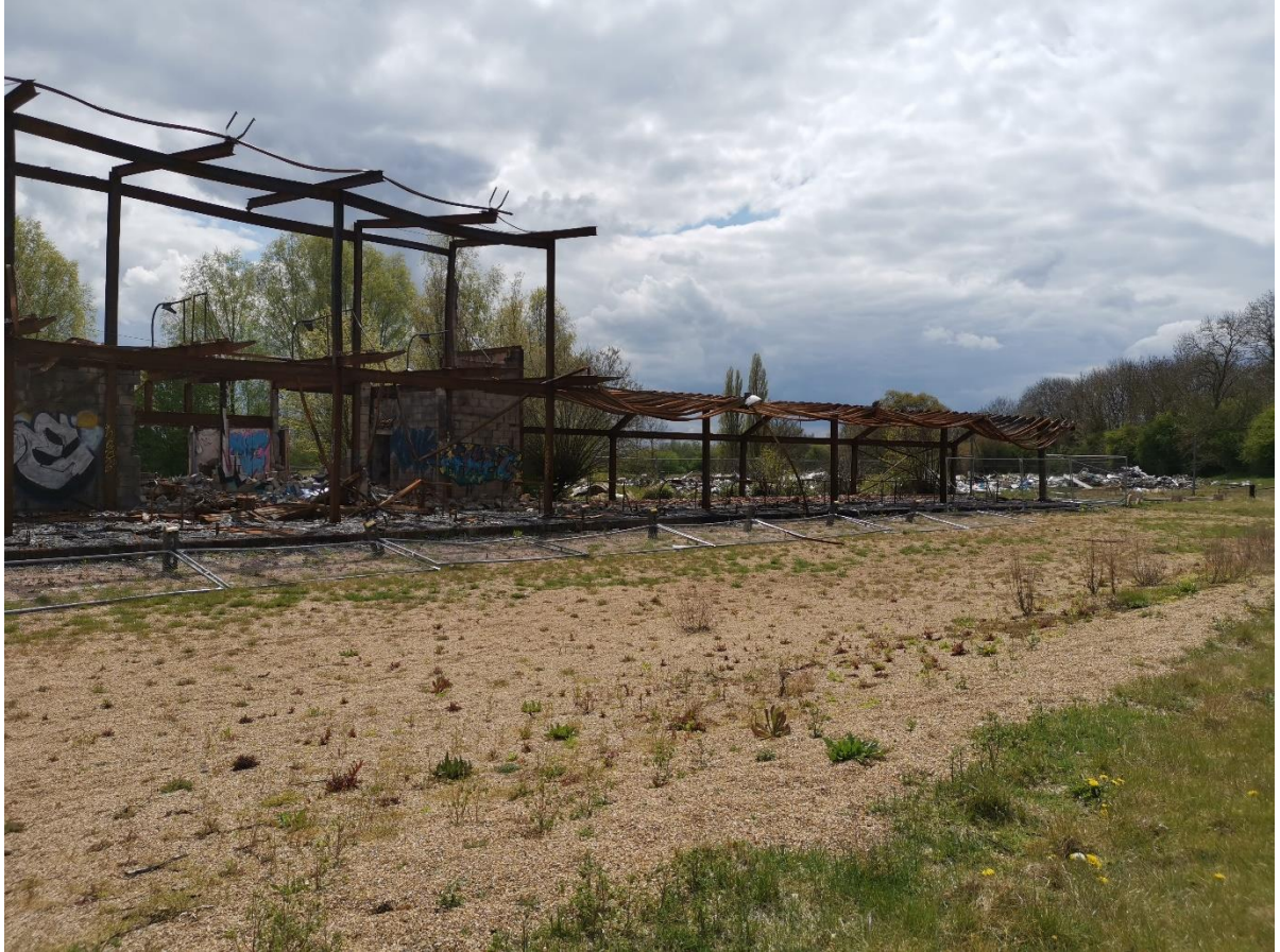
Figure 16: Northern side of remaining structure on site
