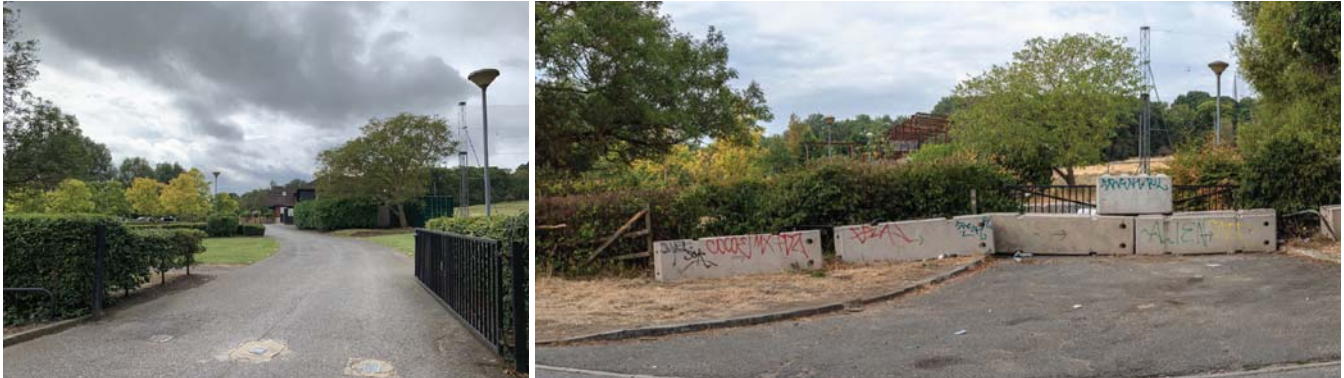
Figure 20 – Photo on the Left before the fire and on the right after the fire.
