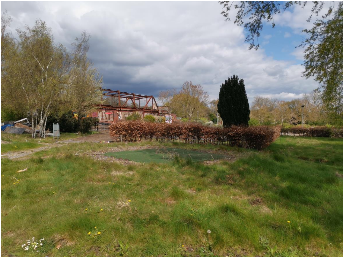
Above: View of the remaining structure from the south
