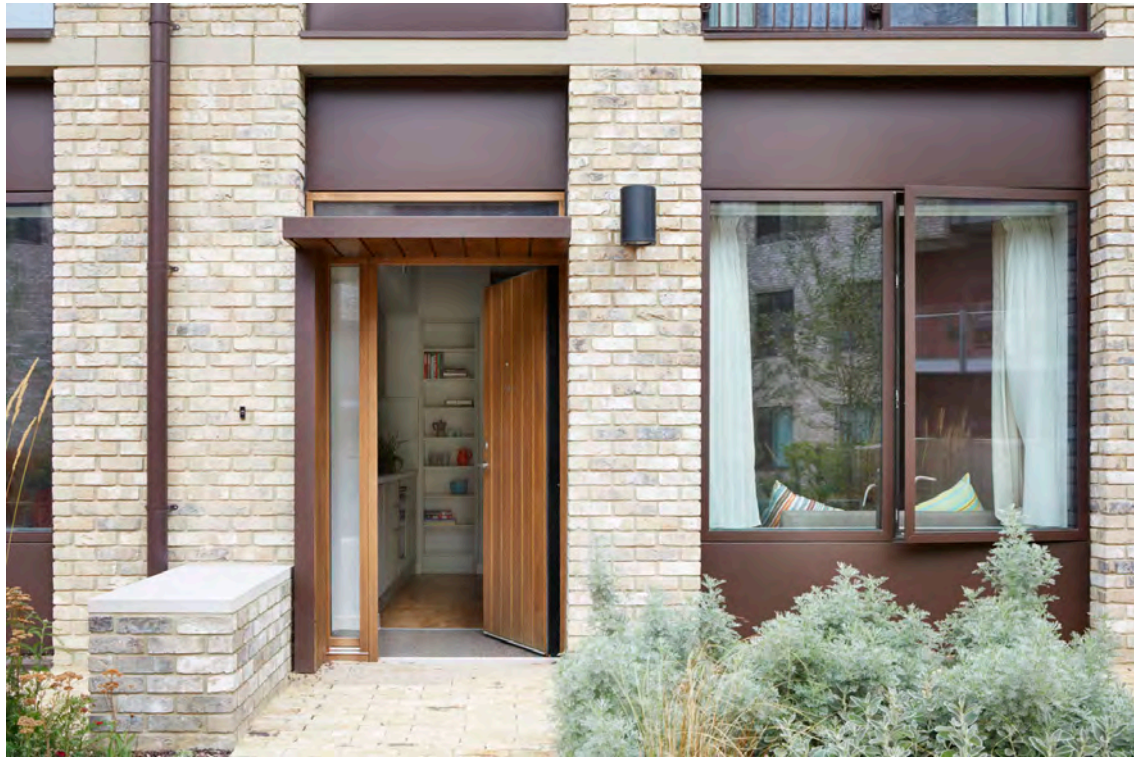
Provide shelter to entrances and threshold spaces ●
