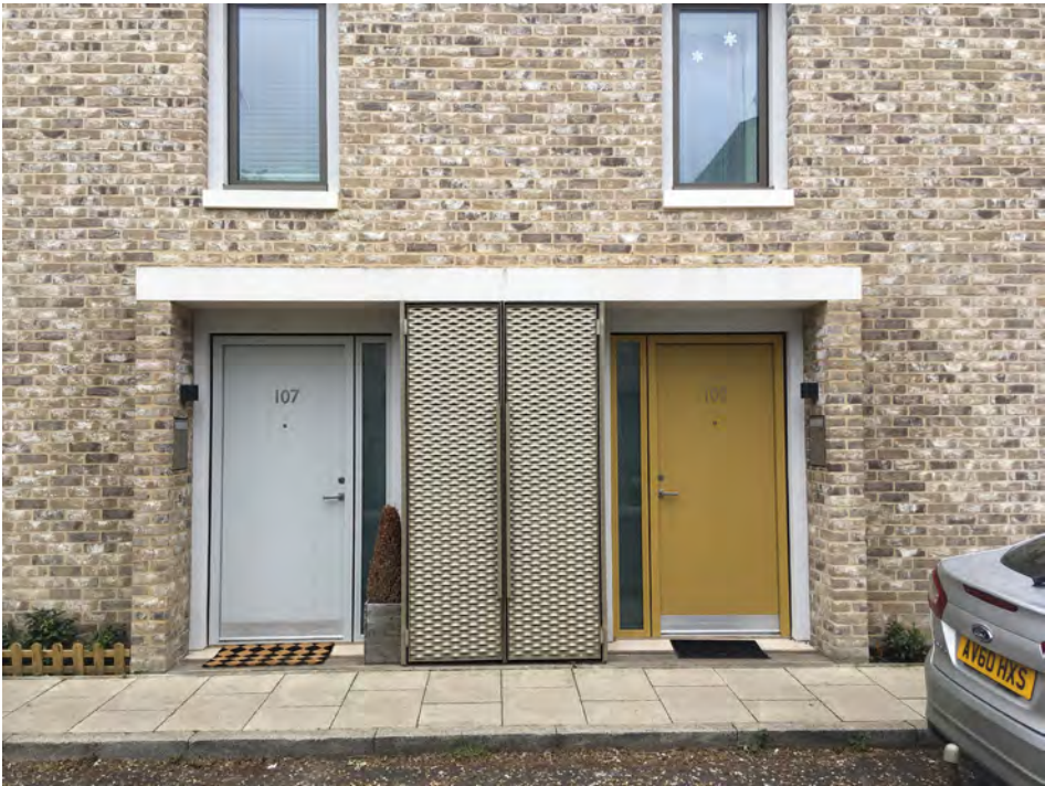
Example of service meters being located externally alongside entrance
