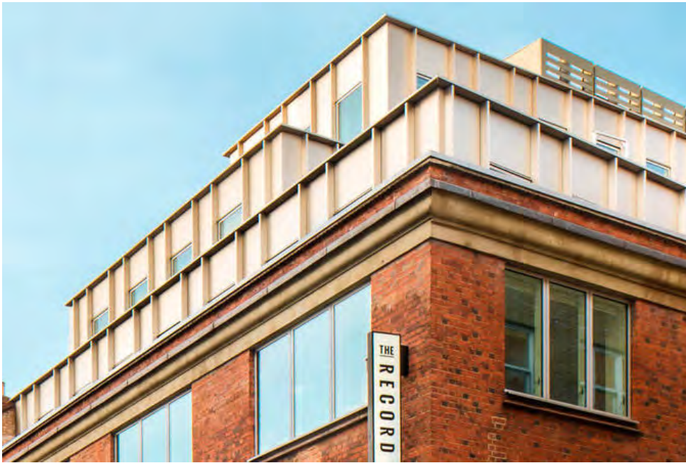
An upper level setback can be distinguished with a different material choice ●
