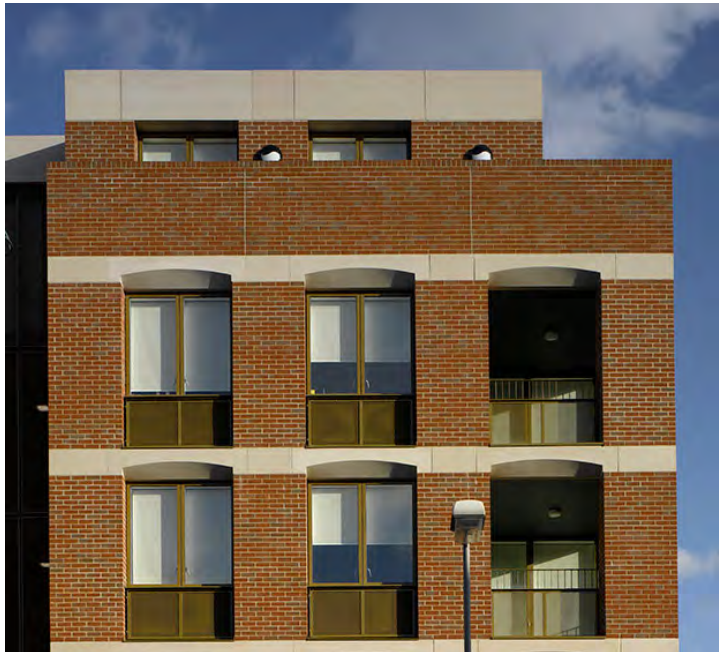
An upper level parapet used with a setback should be solid and use the material of the main facade ●
