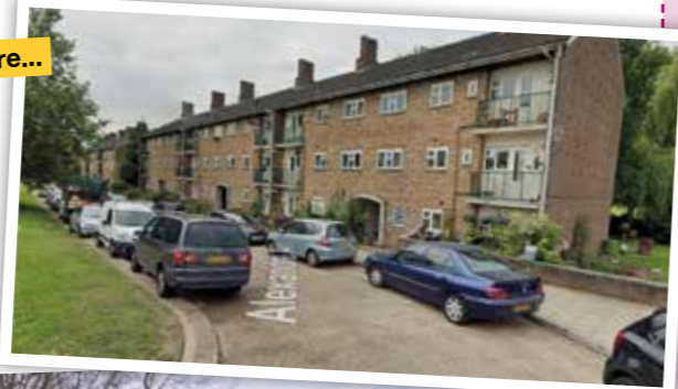
...after, showing the widened access road
