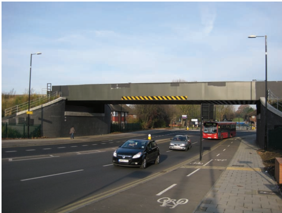
Picture 5 Petts Hill Bridge
