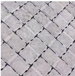
Non-Permeable Block Paving
