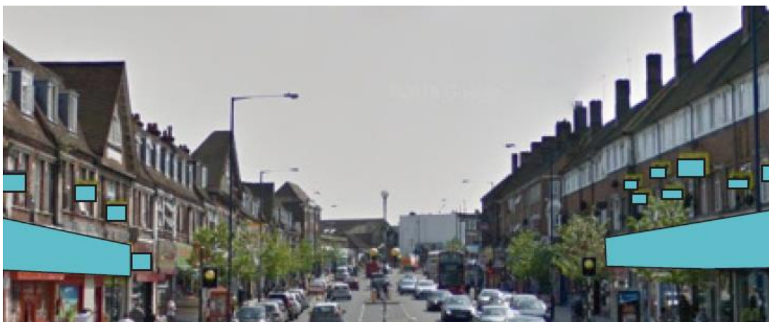
Figure 36 highlight of signs inappropriately placed cover the pedestrian visual field
