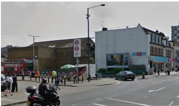
Figure 19 Inactive but visible flank walls
