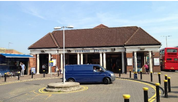
Figure 20 Forecourt to the Station
