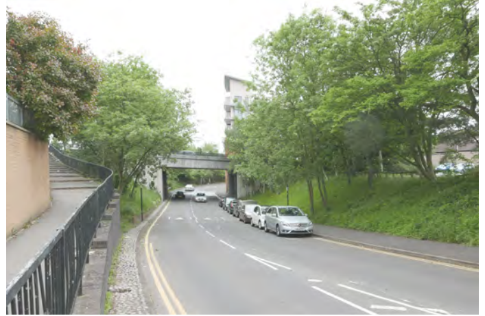
2. Bridge over Marlborough Hill is lacking active frontage but does have mature trees which are an asset.
