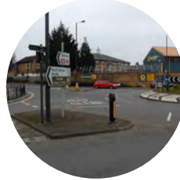
Palmerston Road Roundabout Poor pedestrian environment around roundabout with badly aligned crossing and kerb lines.
