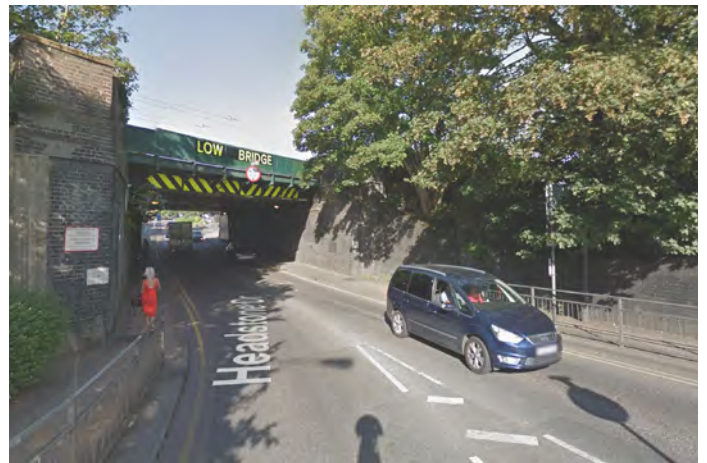
4. Low bridge underpass below rail lines.
