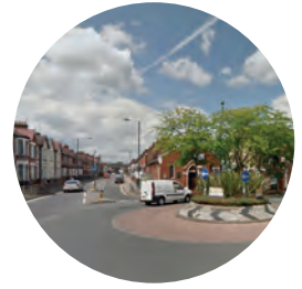
Masons Ave Roundabout Poor pedestrian environment around roundabout with badly aligned crossing and kerb lines.
