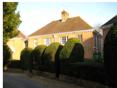
Picture 2.11 Hipped roofs and centrally located chimneys
