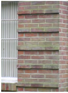
Picture 9.25 Projecting bricks
