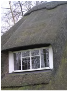
Picture 9.31 Thatch roof
