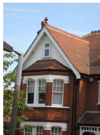
Picture 4.30 Decorative clay pinnacles and ridge tiles, as well as recessed brick aprons
