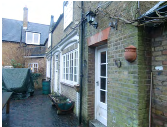
Picture 1.27 Original recessed doorway with gauged brick arch above - mirrored on the other side
