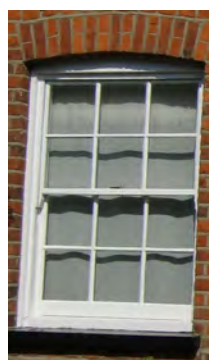
Picture 2.89 Six over six pane timber sash window
