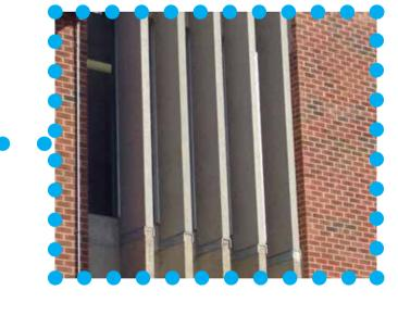
South facing elevation designed to mitigate over looking issues by diffusing views from windows through the use of fins or louvers
