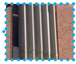
South facing elevation designed to mitigate over looking issues by diffusing views from windows through the use of fins or louvers
