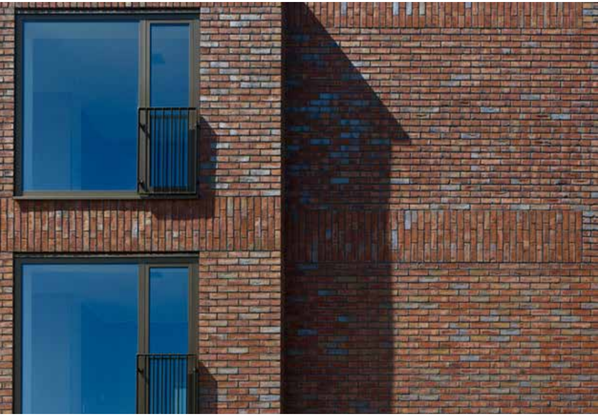
Horizontal banding with vertical stretcher bond
