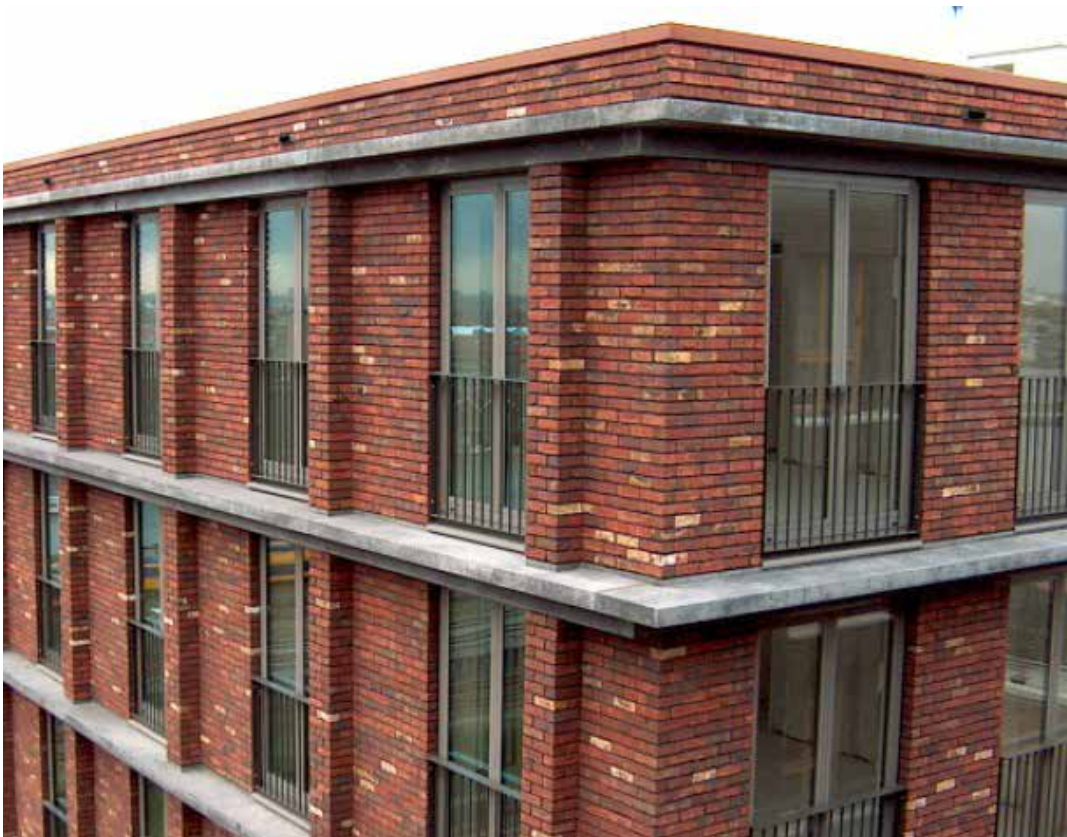
Projecting concrete floor plate banding
