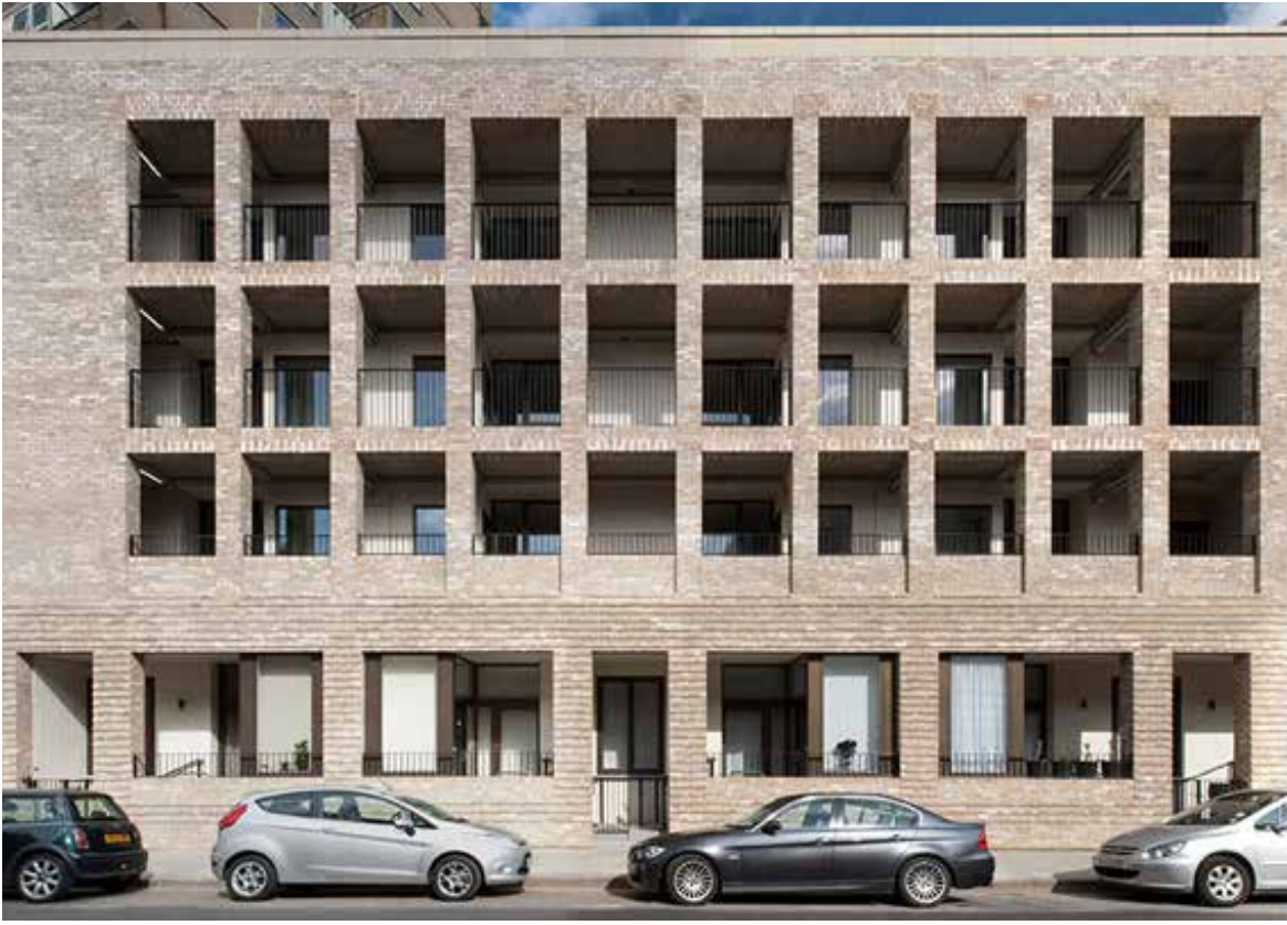
Inset deck access with colonnade of brick piers
