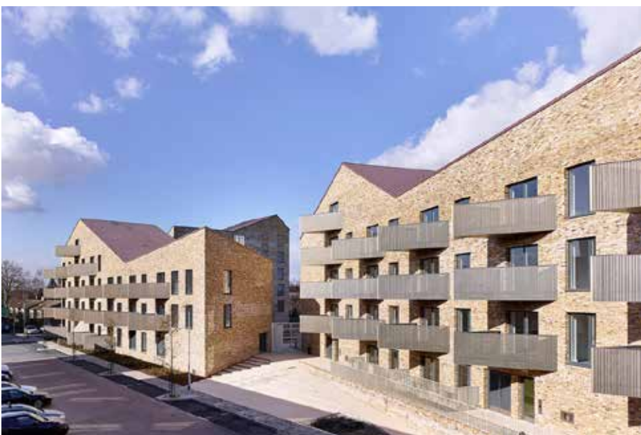
Folding roofscape with standing seam metal roof
