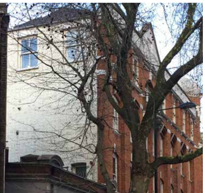
Red brick outer skin 'crust' with a white brick face for the 'core' courtyard skins
