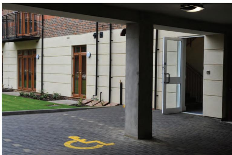
**4.30** **Negotiating the entrance door** *Ensure that the clear opening, approach space and threshold are suitable for use by a person using a wheelchair.*
